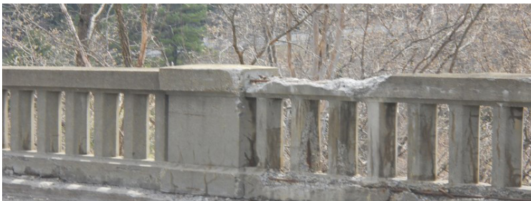
Existing Bridge Rail
